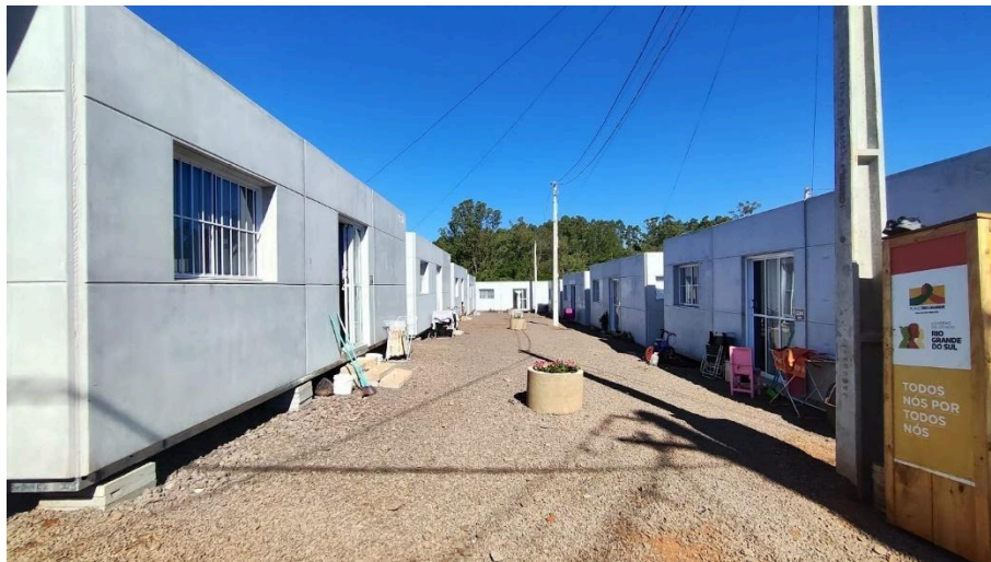
Plate 2. Housing installation in Estrela - RS (Source: Author, 2024)
